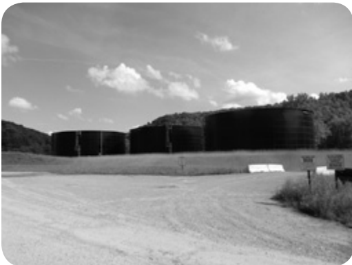
A company just getting established in Doddridge County has prepared for huge volumes of flowback water from its Marcellus fracking wells. These 3 huge tanks will hold about 6 million gallons of flowback each. They are open and liquids are allowed to come within a foot of the top. (Photo: John Wagner)
