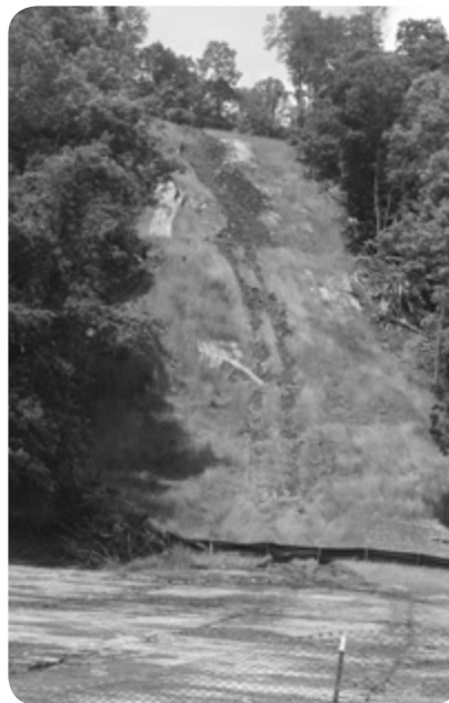
The county’s steep hillsides and creek bottoms are laced with gas pipelines, often from two or three companies in the same cut. The pipeline cuts are often badly eroded and cause significant damage when they cross streams. (Photo: Peggy Wert)
